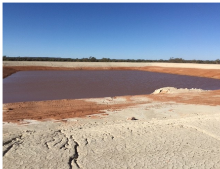
Tullanora Dam, Durham Downs Station
