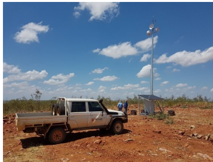
Digital UHF - Hughes Repeater, Ruby Plains Station
